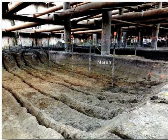
View of Freshwater Marsh Deposits Overlying Colma Sand Exposed near 2nd Street to the North
